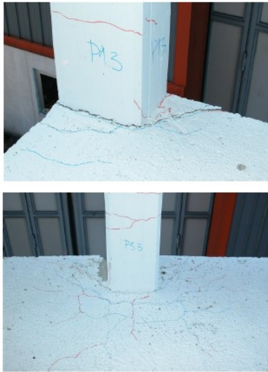
Figure 56. Floor 2 (above): details of cracking around columns P1 and P3
