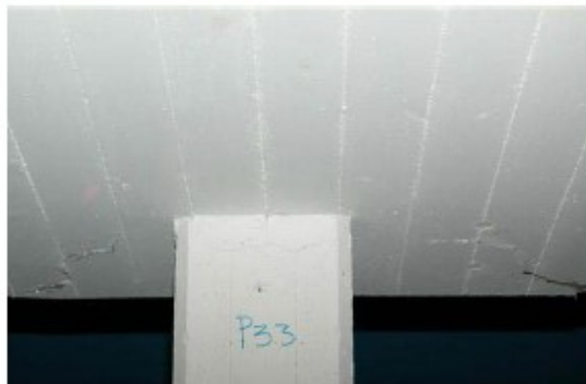
Figure 24. Floor 3 (below): slab crack detail around the perimeter of column P3
